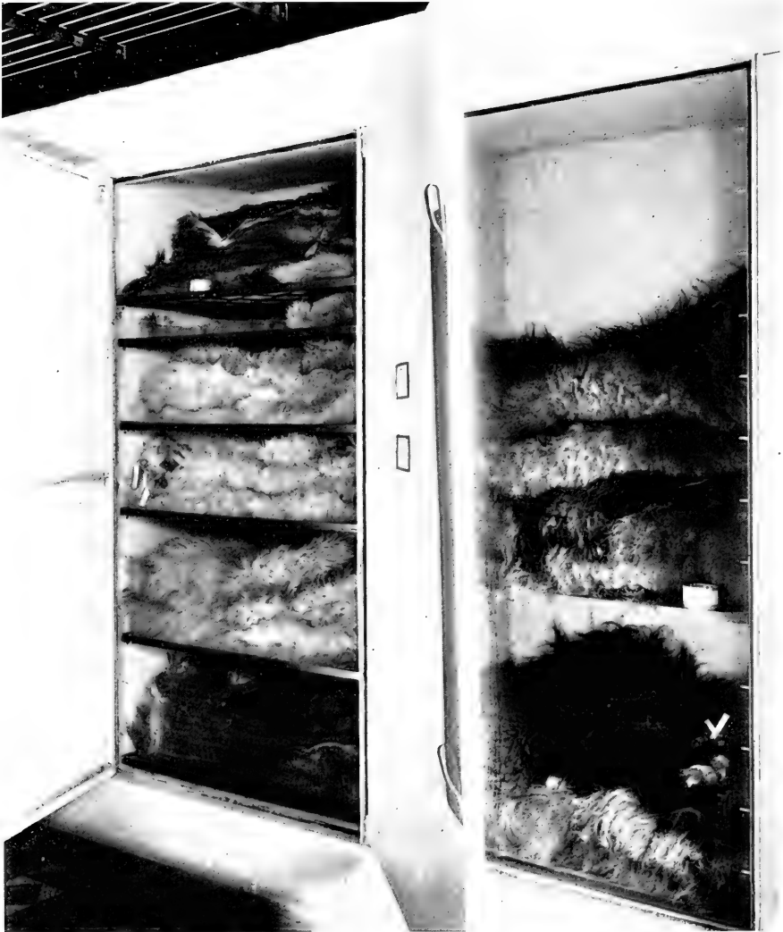
Fireproof storage cases built solidly into the wall. Backs and sides are of cement, doors of iron, trays of woven iron wire. An open can of carbon disulphide protects from insects
